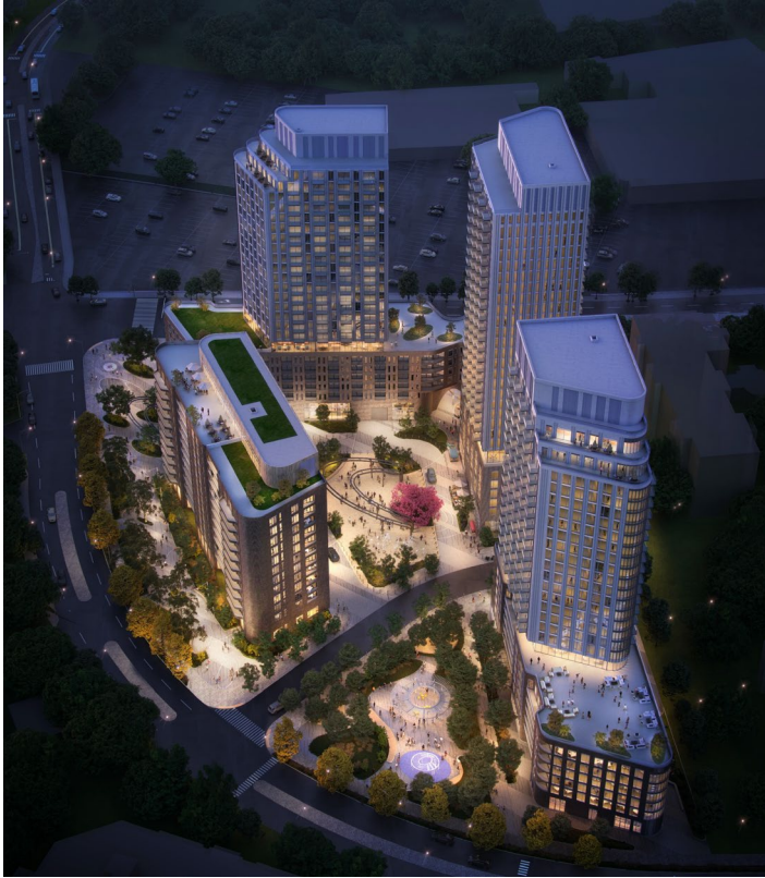
AERIAL VIEW FROM THE SOUTH-EAST CORNER
